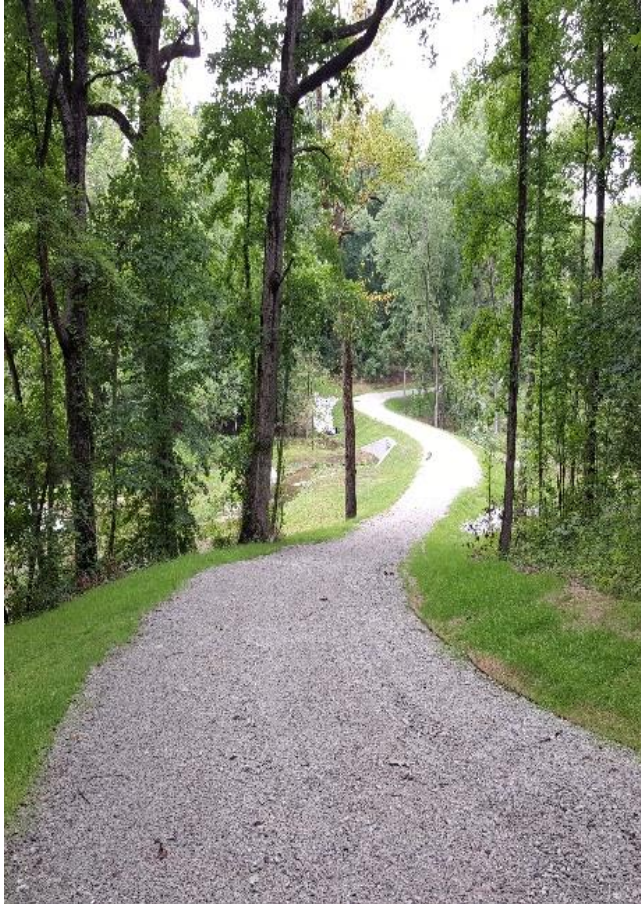
Riverside Stormwater Greenway – a section of the Appomattox River Trail
